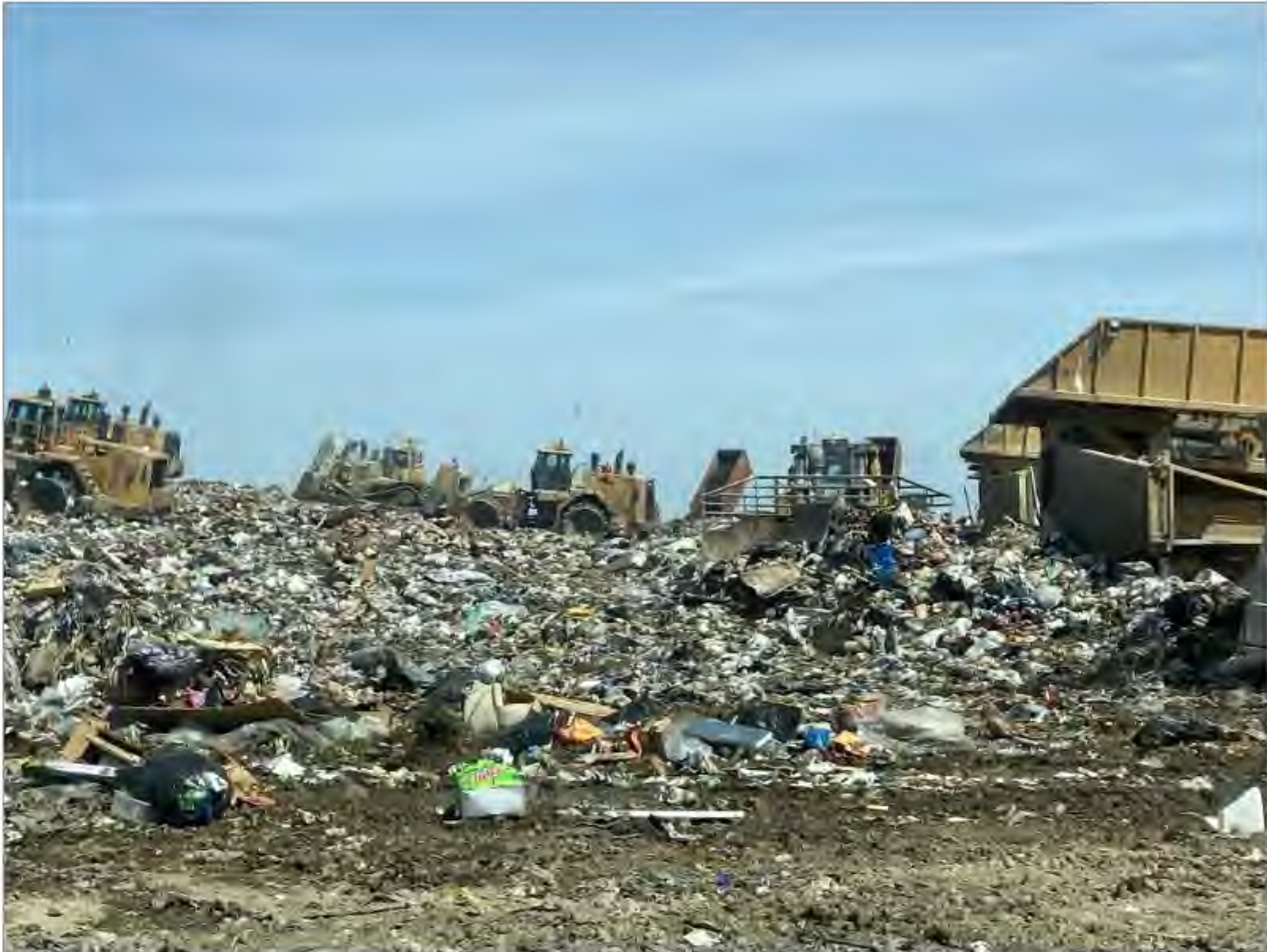
Working face of an active landfill
